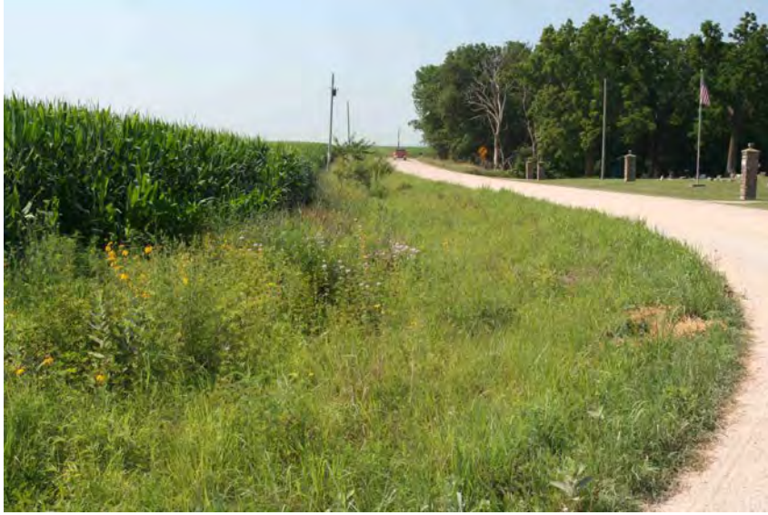
Figure 1. First assessed hydroseeded ROW site in Sac County.
