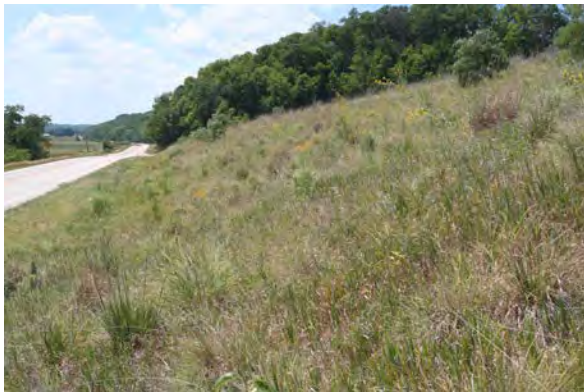
Figure 1. First assessed hydroseeded ROW site in Des Moines County.
