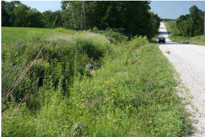
Figure 1. First assessed hydroseeded ROW site in Hardin Co.
